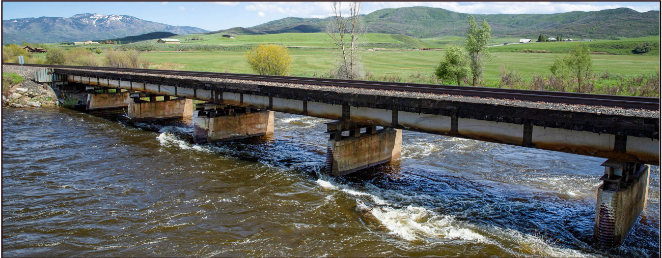
A view of the railroad bridge at RM 194.4, as seen from the river right shore at about 2,000 cfs. A submerged log obstructs the closest channel between the abutments, while another tangle of wood is hung up on the third abutment from the left.
